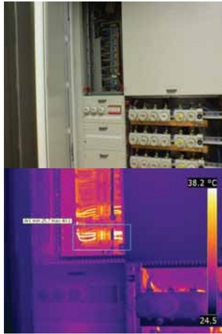
Although these output terminals are definitely hot, the measured temperatures are normal for this kind of load.
