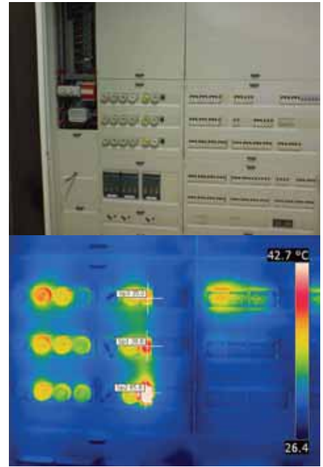
This thermal image shows that the work load during operation is not distributed evenly among the fuse boxes.
